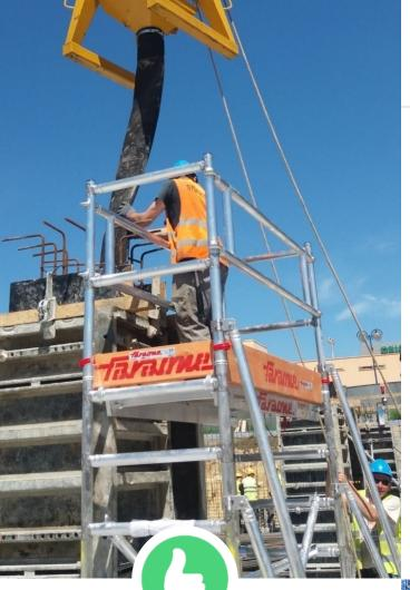
The use of complete scaffolding during carpentry and reinforcement works significantly reduces the risk of falling from a height.
