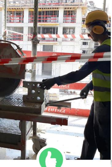
Processing materials generates physical hazards. Wet cutting and PPE's, such as safety glasses and hearing protectors, protect workers from their negative effects.
