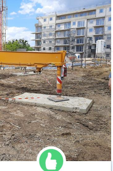
Spreader pads provided under outriggers guarantee a sufficient stability of vehicle and prevent from tipping
