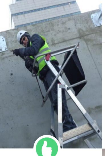
Platfrom ladders enables to perform works with both hands, also such ladders are equipped with guardrails around platform.
