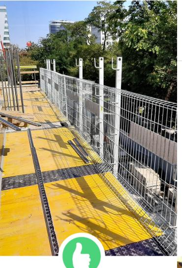
Full system edge protection (mesh panels) is easier to install and provides more effective protection against falling down.
