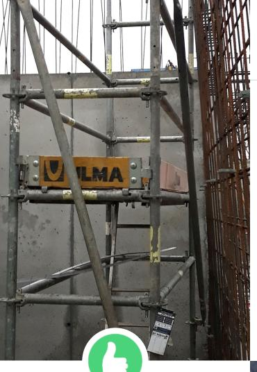
Complete scaffolding with required guardrails, toeboards and scaff-tag.
