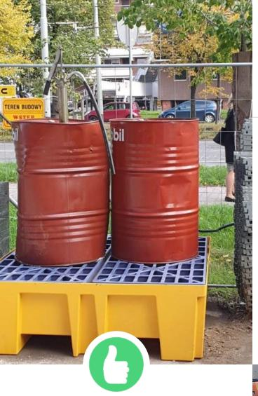
Properly stored chemicals on anti-spillage tanks - in case of leakages can avoid soil spillage.
