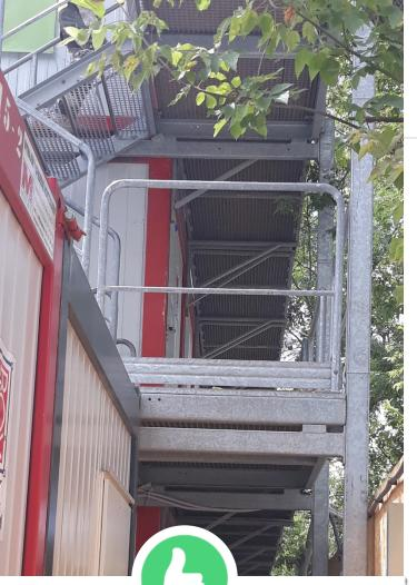
Proper system platforms, stairs and guardails at site welfare containers.
