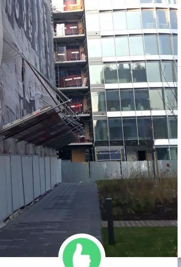
Roofing within hazardous zones reduces the risk of falling objects on the ground.
